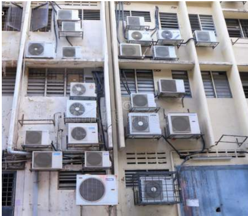
Figure 25 A common site in Malaysian cities: external walls covered with air-con units.
